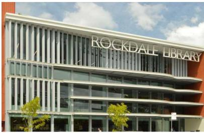
CVS Shadelite Ellipsoid Screens can be coated in a range of different finishes to suite specific requirements, including warranty and custom colour powder coat through to bright coloured anodising.
