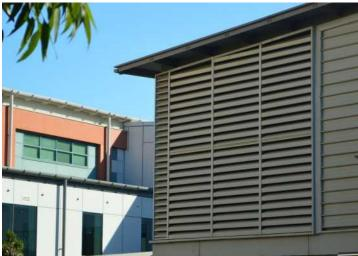
CVS Freeflow Acoustic Louvres can be coated in a range of different finishes to suite specific requirements, including warranty and custom colour powder coat through to bright coloured anodising.
